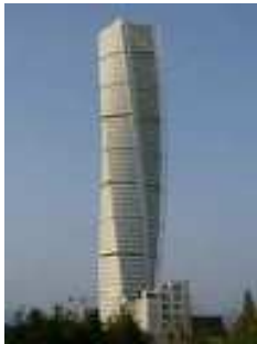
Figure 3: The Turning Torso (2000-2005) in Malmo by Santiago Calatrava [2,3]
