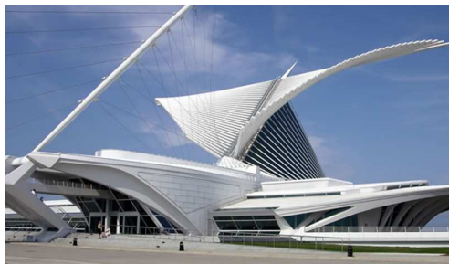
Rys.1 Milwaukee Art. Museum projektu Santiago Calatravy, stan Wisconsin, USA.
