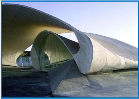
Fig.2. A bus stop in Casar deCaceres in Spain.
