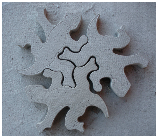
Figure 13: Concrete paving designed on the equilateral triangle basis (photo: E. Koźniewski)
