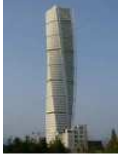
Figure 3: The Turning Torso (2000-2005) in Malmö by Santiago Calatrava [2,3]
